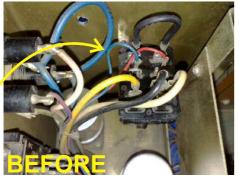
To disable BE motor only at time out, remove BLUE wire from BE relay (coil) and connect to one of the new PURPLE wires. Connect the other new PURPLE wire to the coil of the BE Relay where the original BLUE wire came from.
